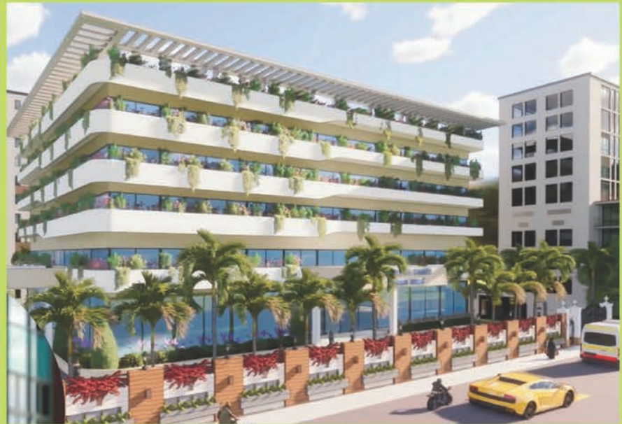
New Goutami Institute to be constructed 2024
