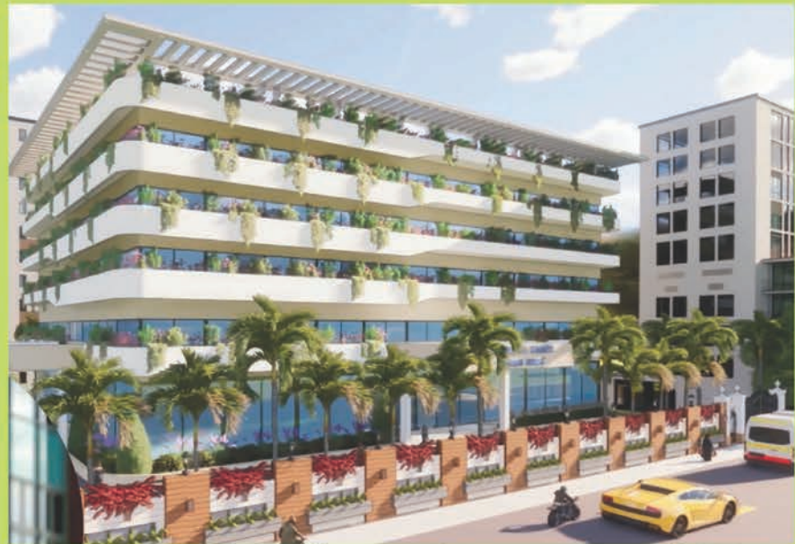
New Goutami Institute to be constructed 2024
