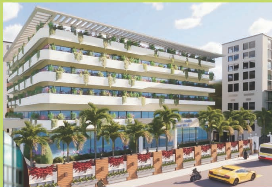
New Goutami Institute to be constructed 2024
